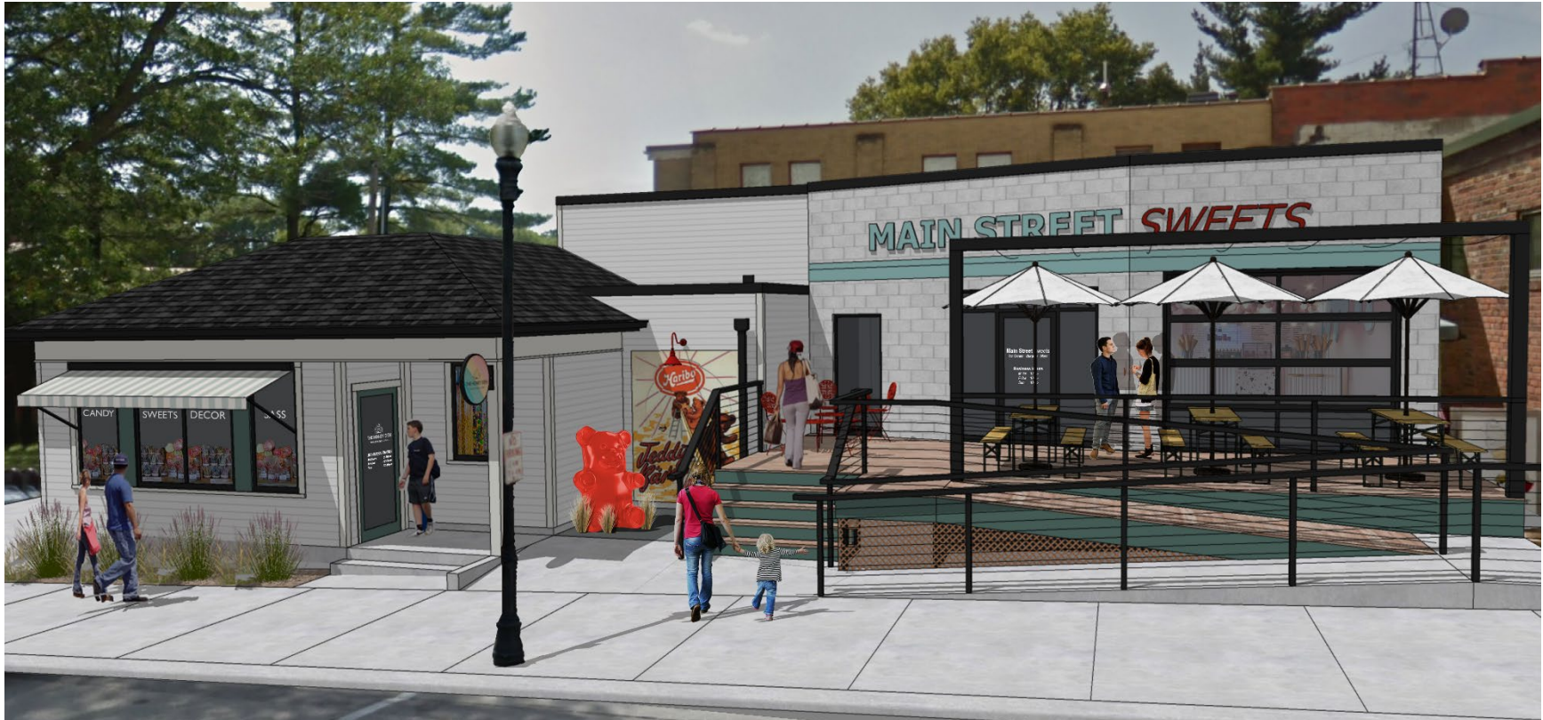
Option A: Concept rendering from Main Street showing addition with covered corner entry, and second addition with flat roof and parapet. The exterior cladding is removed from the Main Street Sweets building and updated windows.
