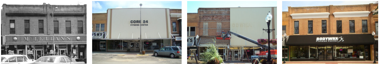
Rehabilitation of a historic building in downtown Washington included removal of an inappropriate, non-historic slipcover.
