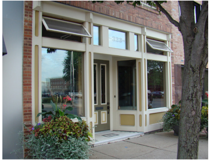
Operable transoms are integrated into this reconstructed storefront for added light and ventilation.
