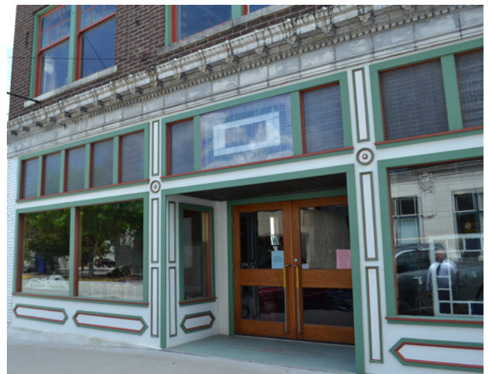
This reconstructed wood storefront contains traditional elements, highlighted by a three-tone color scheme.
