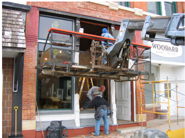
New storefront window frames are constructed between historic cast iron columns.
