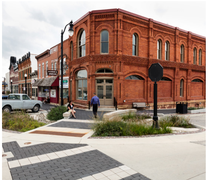
Permeable pavers and bump outs at intersections provide both safety and sustainability improvements in West Union.
