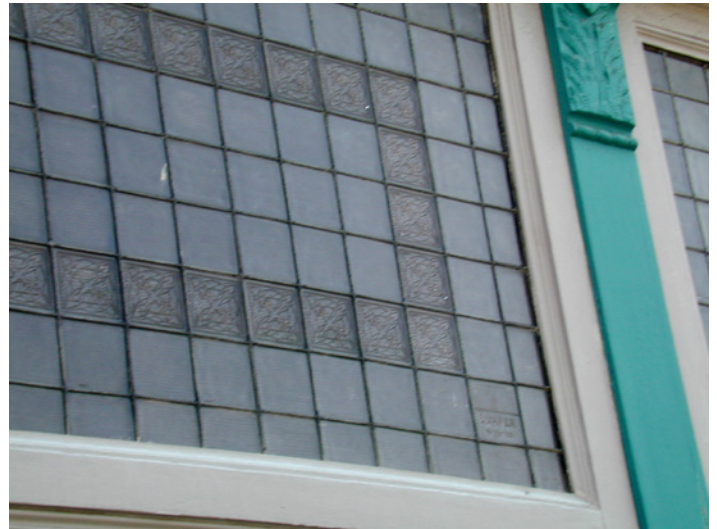
Prism glass was often used in transoms to direct light further into deep traditional commercial buildings.
