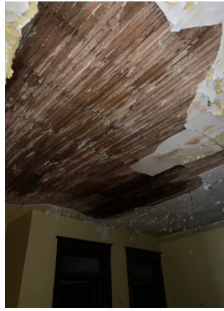
Deferred roof maintenance and improper downspouts can cause significant issues due to water infiltration.
