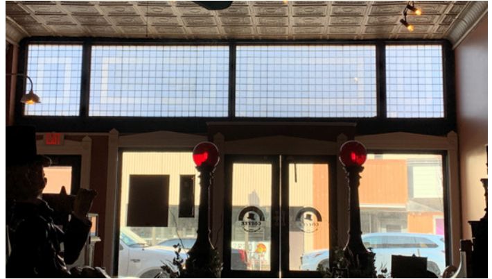
These prism glass transom windows maximize natural light and enhance the interior space.
