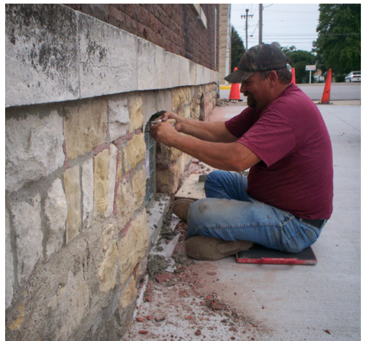
Mortar used for repointing should match original mortar in color, texture, and strength to protect historic masonry.
