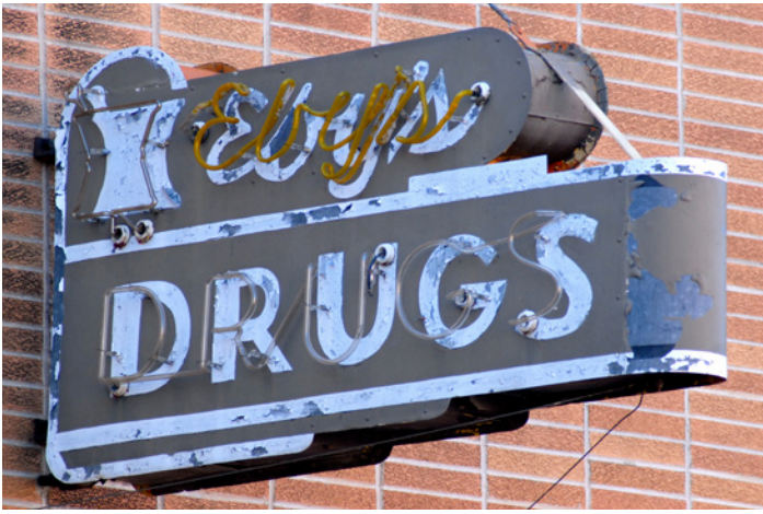
Historic neon signage can be retained and restored or retrofitted to reflect new businesses.
