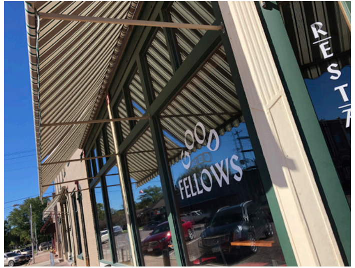
This operable awning allows shade when needed but can also be raised to reveal the transom windows.
