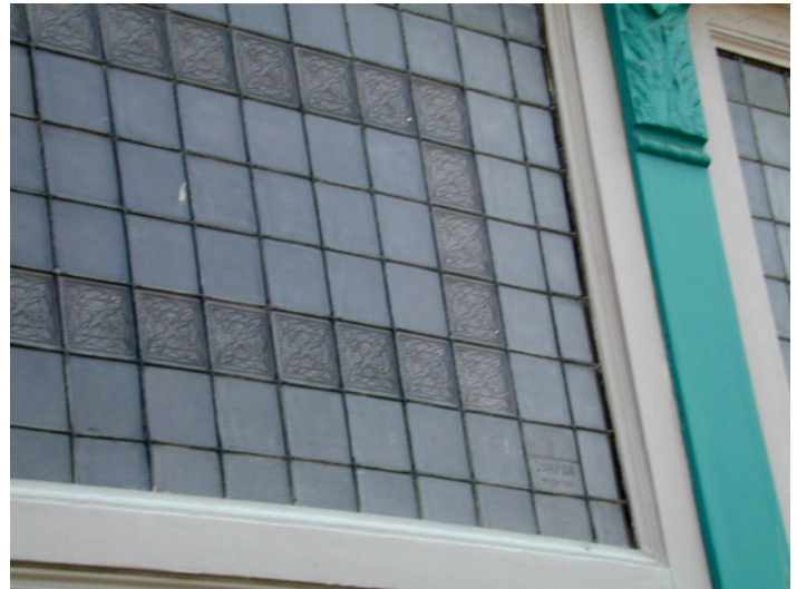
Prism glass was often used in transoms to direct light further into deep traditional commercial buildings.
