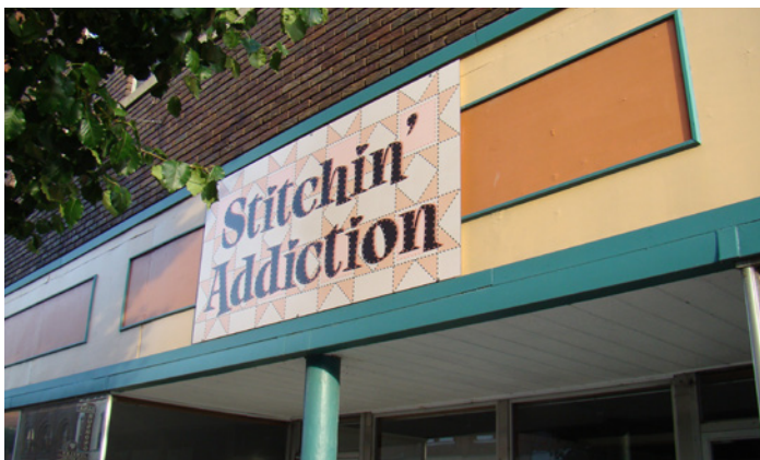
This sign disregards the proportion of the sign panel. A horizontal sign within the orange area would be appropriate.
