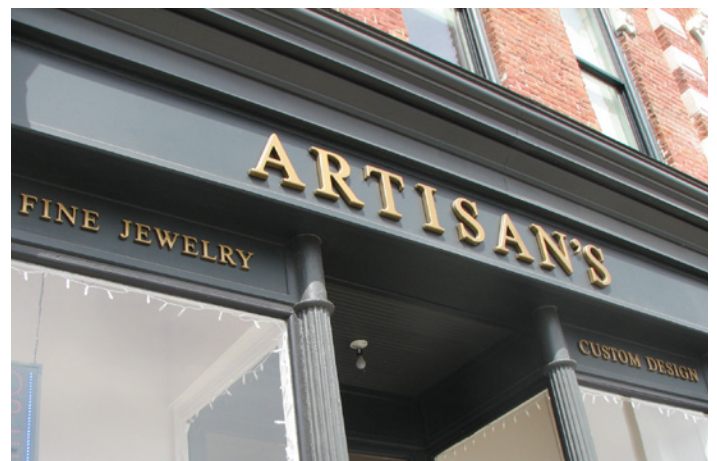
This individually mounted letter signage fits well within the storefront cornice and contributes to a traditional, elegant look.
