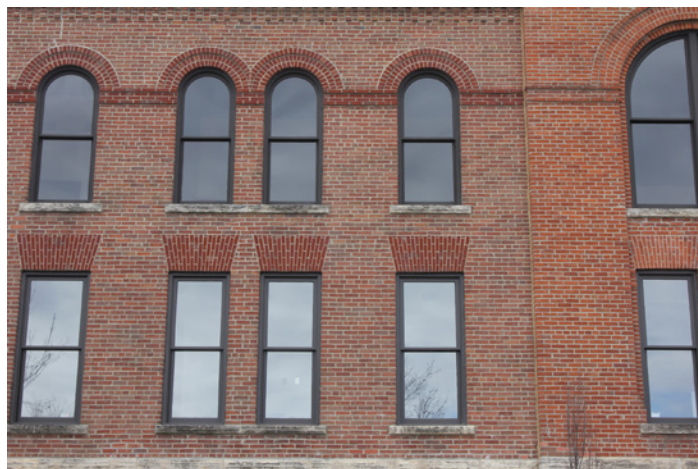
Appropriate window replacements fill the entire opening.
