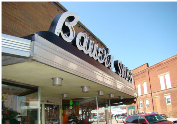
This integrated canopy signage is a character-defining feature of this mid-century building.
