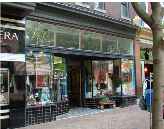
This intact historic storefront features a stepped recessed entry, bulkhead tile, and thin metal window frames.
