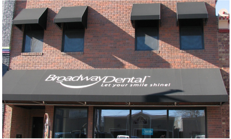
Individual upper story window awnings provide sun shading and coordinate with the storefront awning.
