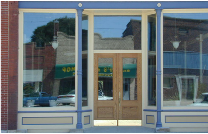
The historic structural columns and lintel were utilized with new wood elements in the restoration of this storefront.
