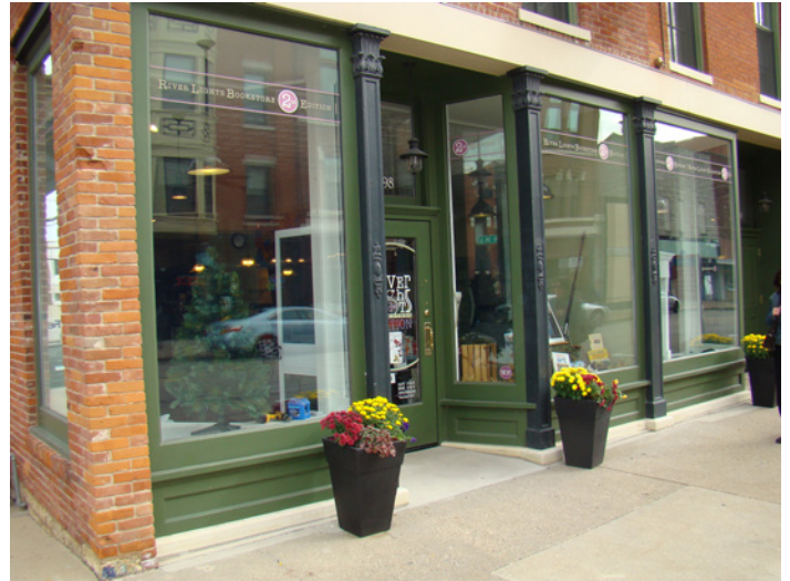
These display windows fill the full height of the original storefront opening in this reconstructed storefront.
