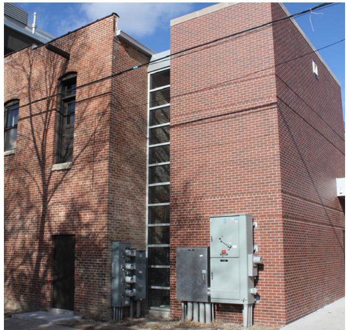
A glass hyphen joins this rear elevator addition to the original building, and distinguishes it from the historic construction.
