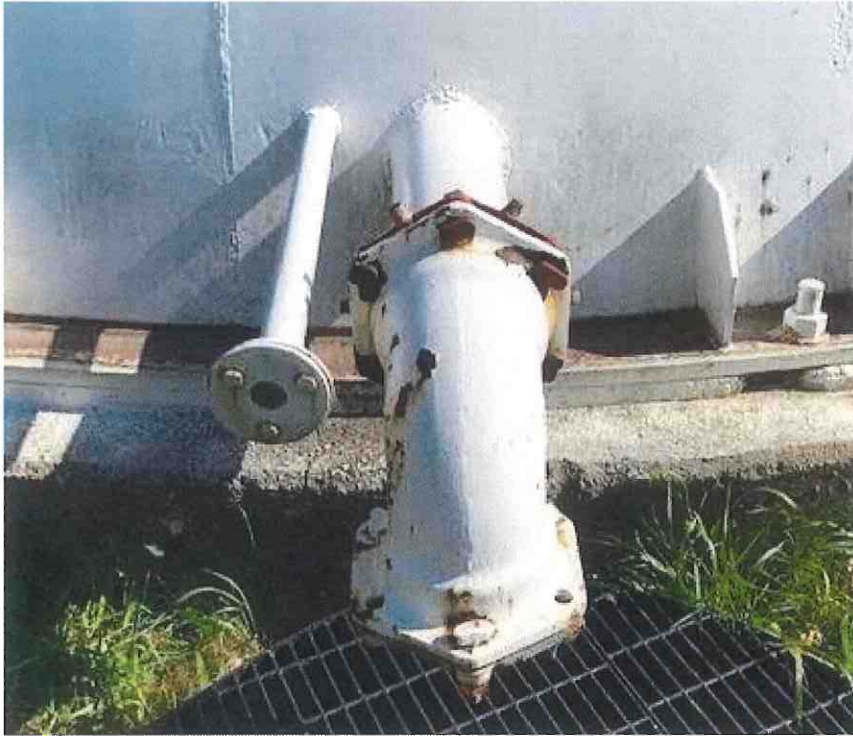
Remove and weld new 90* overflow pipe
