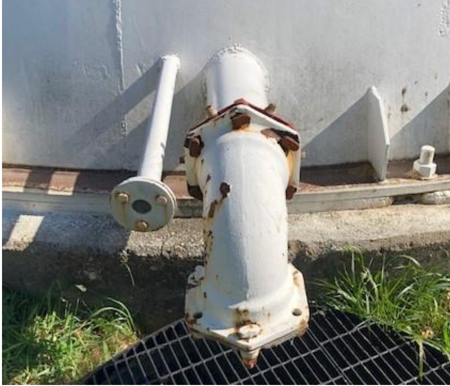
Remove and weld new 90* overflow pipe
