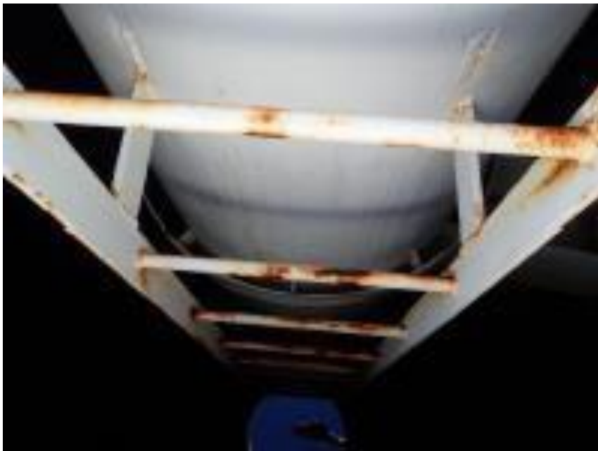
Replace top 5 feet of wet interior ladder
