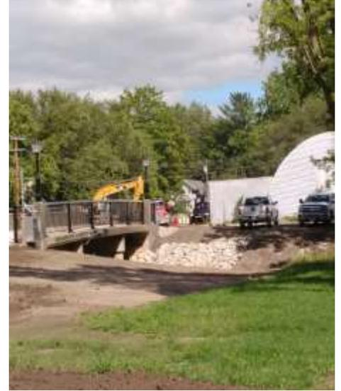
Last week, the contractor began installing the storm sewer and water main on the east side of the bridge. The intersection of 1<sup>st</sup> Street and College Street was also poured.
