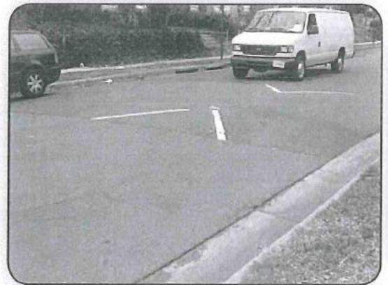
A speed hump is effective at reducing traffic speeds. Generally, speed humps are compatible with snow removal and truck traffic.
