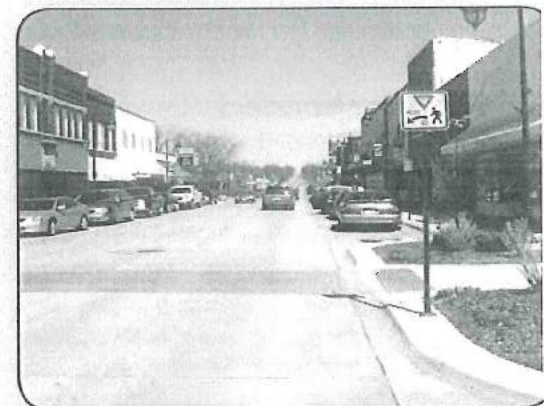
A bump-out in the Delwein downtown area shortens the pedestrian crosswalk and narrows the traffic lane enough to slow cars.
