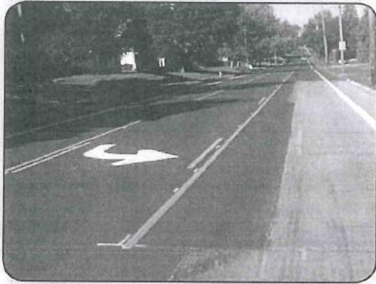
Davenport reconfigured a four-lane road to a three-lane road diet. The center turn lane helps reduce collisions. The remaining space is used for bike lanes.
