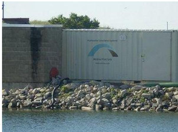
Wastewater Compliance Systems (WCS) and its independent representatives Jim McFarland and Eddie Stewart, of JCI Inc., have been working with the IDNR to prove that communities do not have to abandon their lagoons. Rather, by retrofitting the wastewater lagoons with fixed film bio-reactors, lagoons can, and have shown the ability to nitrify in water temperatures as low 0.4 oC (32.7 oF).
