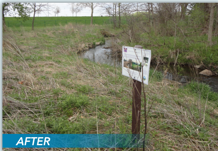
Stream restoration project on Dry Run Creek on the University of Northern Iowa campus, incorporating sloped banks, bank "hides" for fish habitat, and native prairie. The creek withstood the massive rains and floods of 2008, among other high flows. Photos courtesy of Josh Balk.
